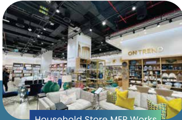
Household Store MEP Works
