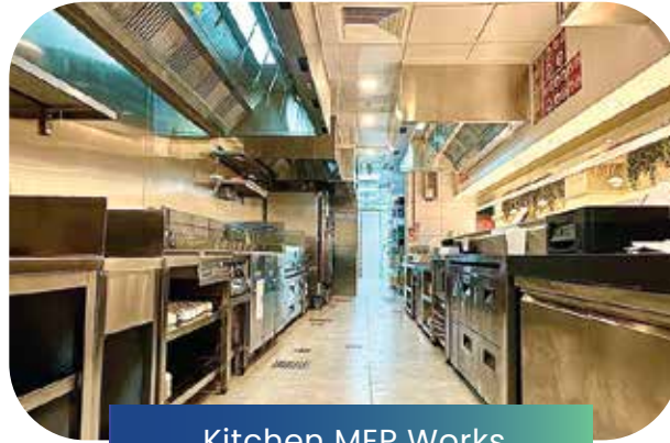
Kitchen MEP Works
