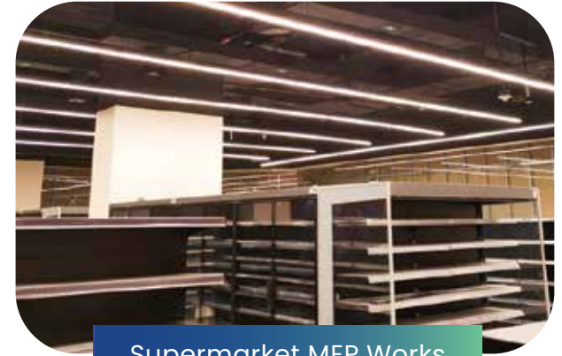
Supermarket MEP Works
